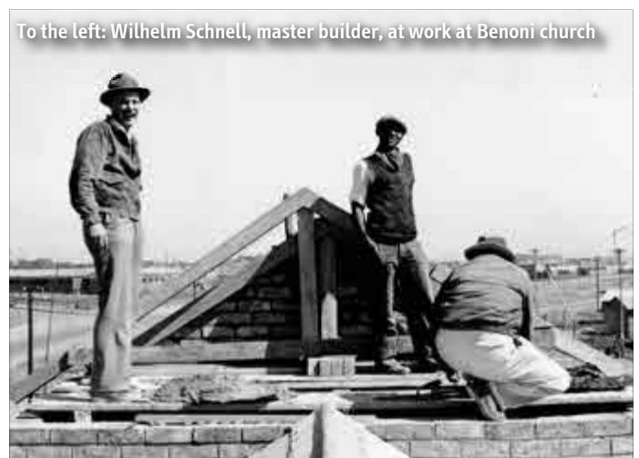
Building the church at Benoni.
